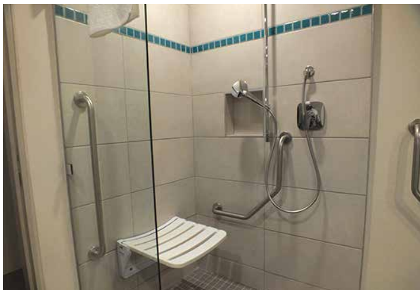
UA roll-in shower in Skukuza Safari Lodge with fold-up shower seat and height-adjustable shower head
